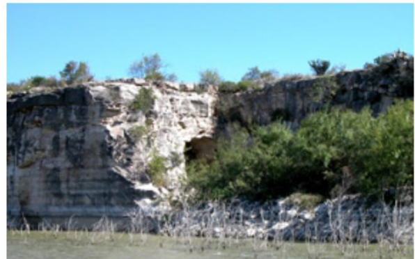
Contemporary photo of historic railroad tunnel
